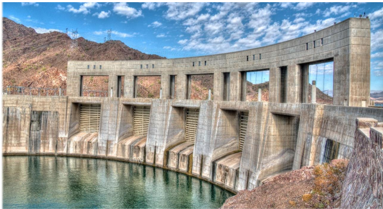
Figure 3.1 Parker Dam at Colorado River
