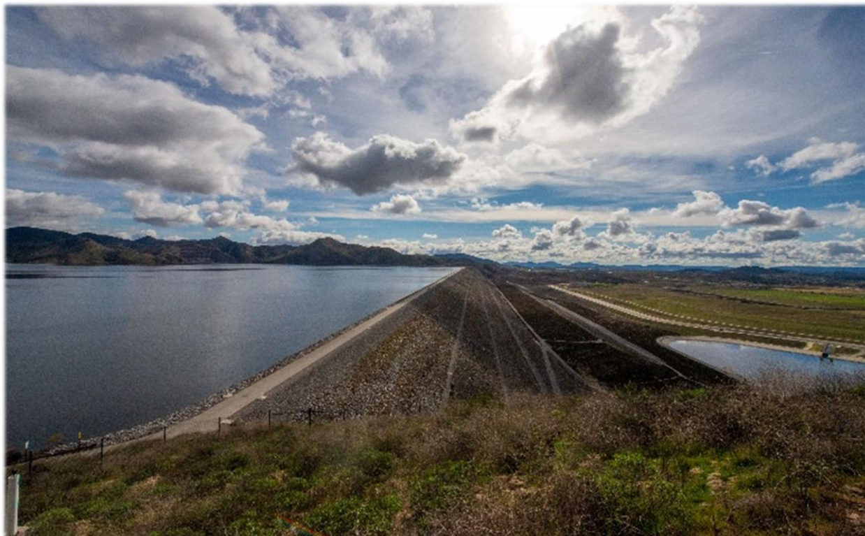
Figure 8.4: MWD's Diamond Valley Lake (Potential Reserves for WSAP Allocations)
