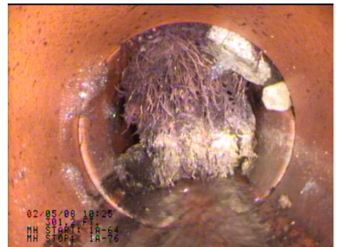
Significant Damage – Major root intrusion. Pipe losing capacity and greatly increased chance of blockage
