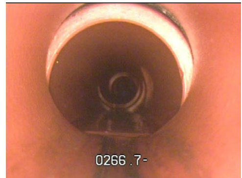
Moderate Damage – large offset that may lead to flow problems. Joint still in tact
