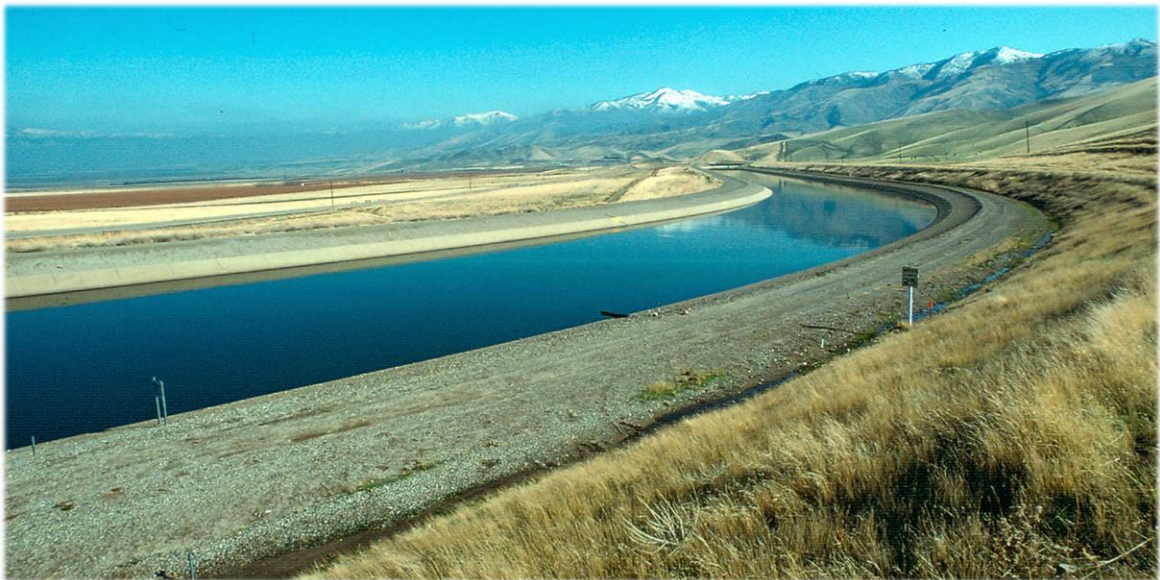
Figure 3.3: California Aqueduct or “SWP”
