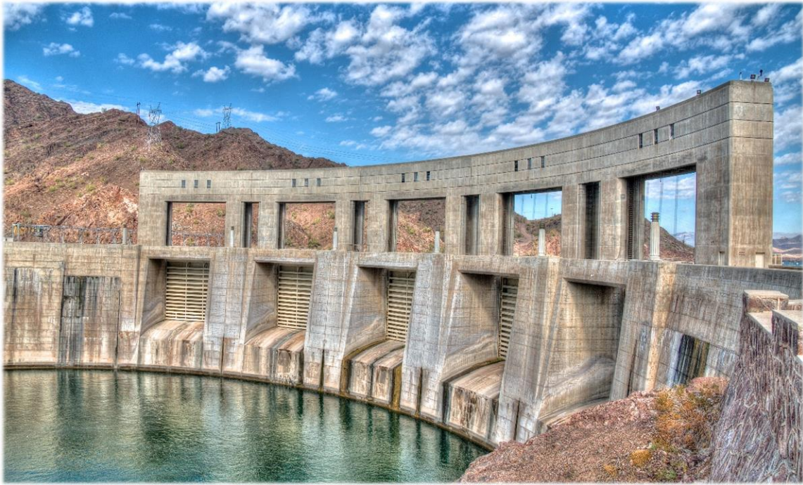
Figure 3.1: Parker Dam at Colorado River
