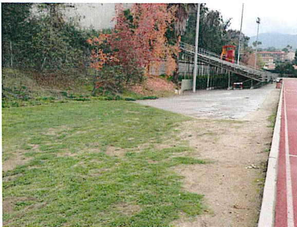
Northwest view of potential MBR site at LCHS partially paved with damaged concrete (Photo Credit: Alex Fagnan, Department of Landscape Architecture, Cal Poly Pomona/2012)
