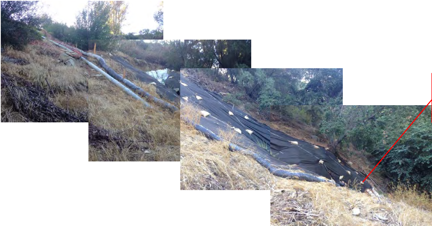
VIEW LOOKING SOUTH AT SLOPE REPAIR.
