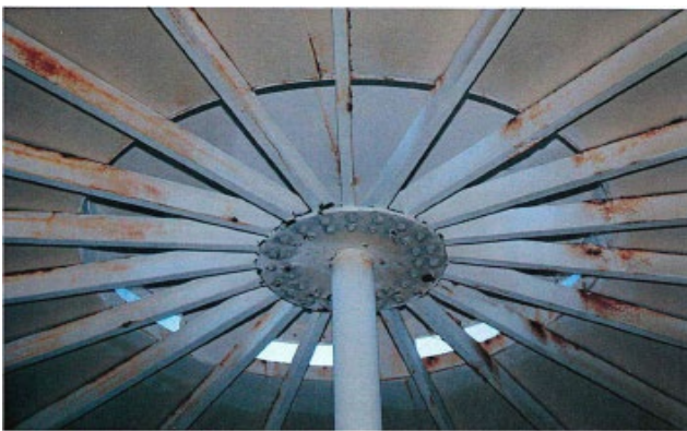
View of underside center vent cover
