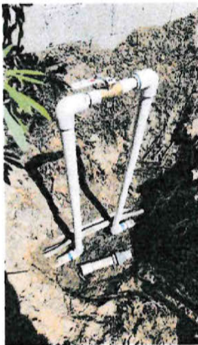
PIC 5. Ball Valve Install
