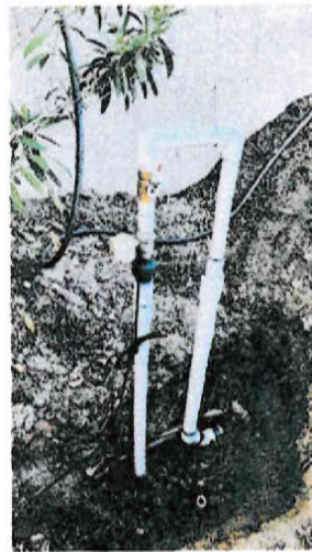
PIC 6. Motorized Valve Install
